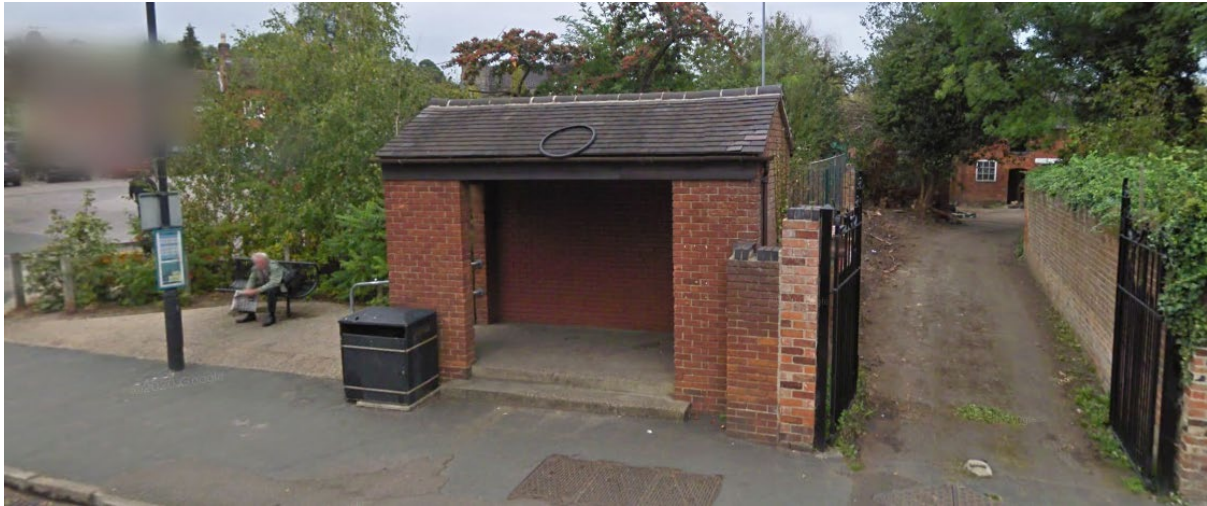
Figure 3: Duke Street Bus Shelter
