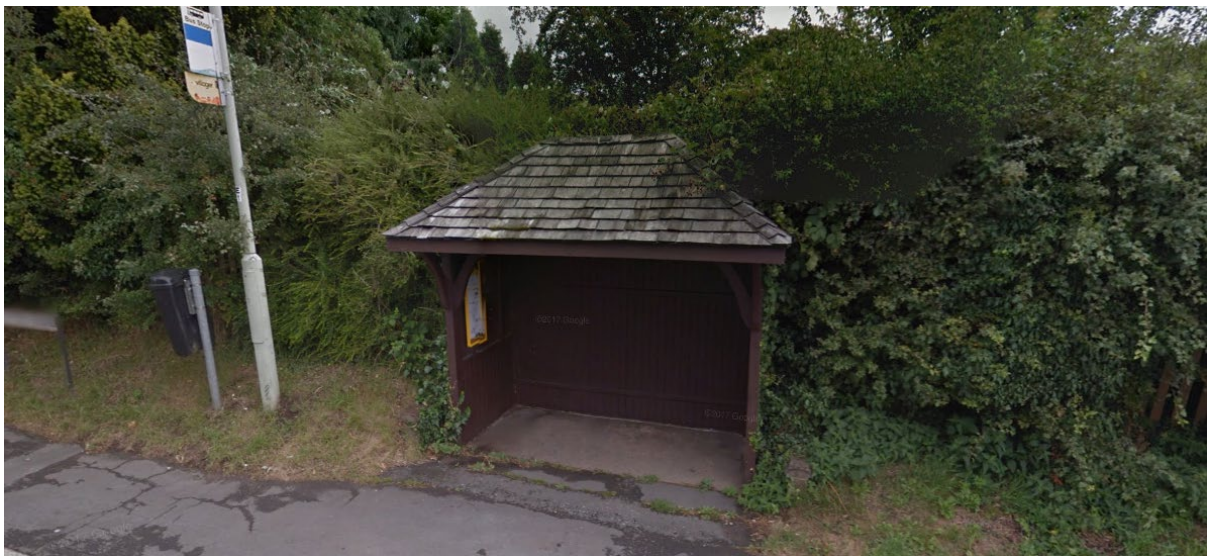
Figure 4: Burton Road Bus Shelter
